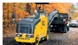
Asphalt milling machines
